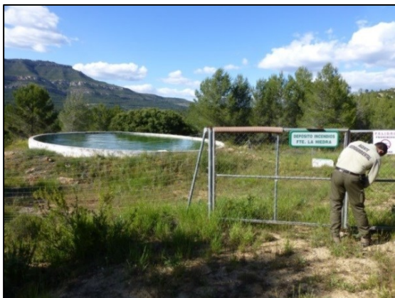
Image 57: Water pond for fire extinction (Nina Lauterburg 2013)
