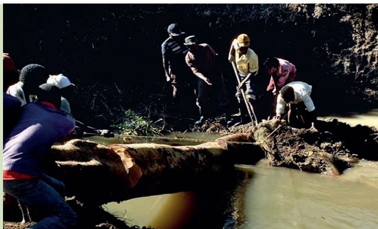
Members of a water user association work together to dismantle an illegal water diversion. Photo: CDE/CETRAD
