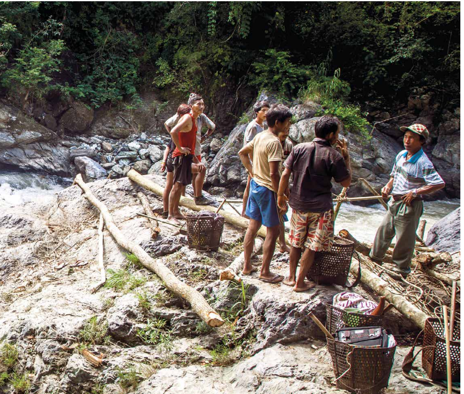
A smallholder fishery in Layshi Township, Northern Myanmar: Villagers are constructing a fishing fence. Photo: Lin Bo Jian
