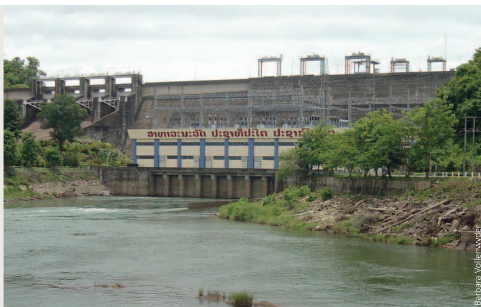
Nam Ngum dam and power station, Lao PDR.
