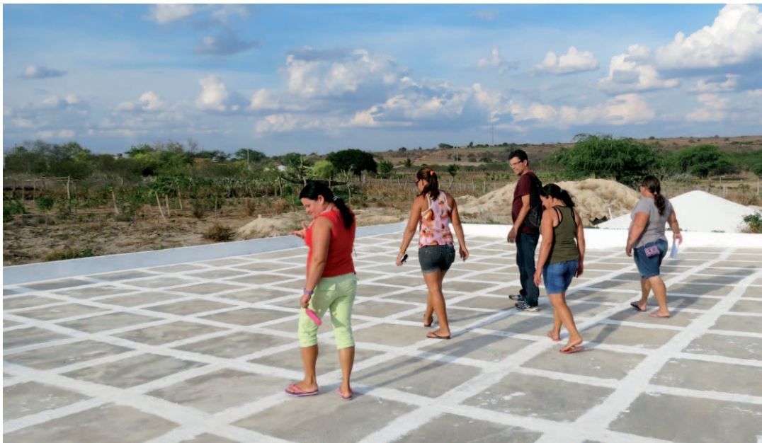
Cement cisterns are constructed for rain water harvesting. © Matheus Alves Zanella
