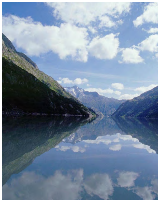
The Grimselsee with a volume of 95 million m 3 is the largest reservoir lake in the Grimsel area. (Photo: KWO)
