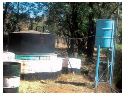
Gas collection tank resting on the concrete-built digester. Pipes / tubes at the top of the gas tank supply the house with methane gas, Botswana. (Reuben Sebugo)
